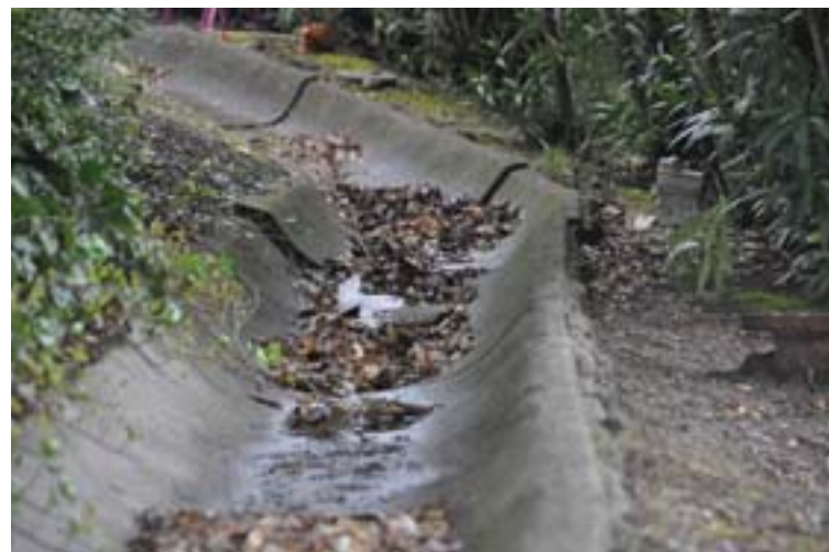
Typical storm drain in a Moraga neighborhood. Photo A. Scheck
